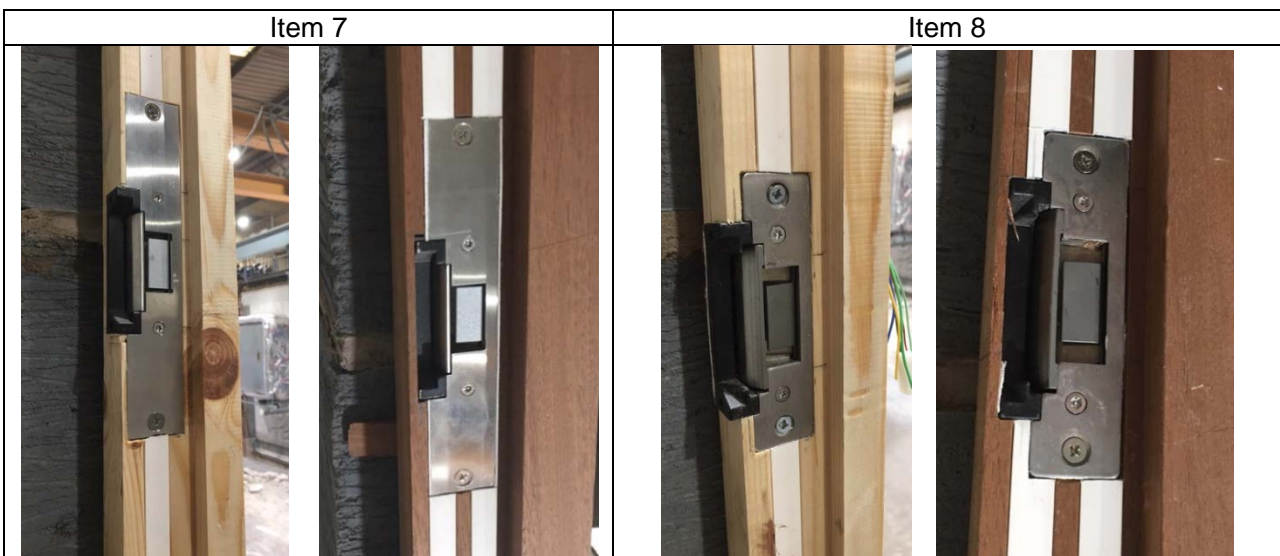
Strike (fail secure) / showing intumescent interruption
